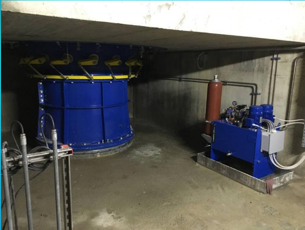
Double regulated Kaplan turbine coupled with PMG
