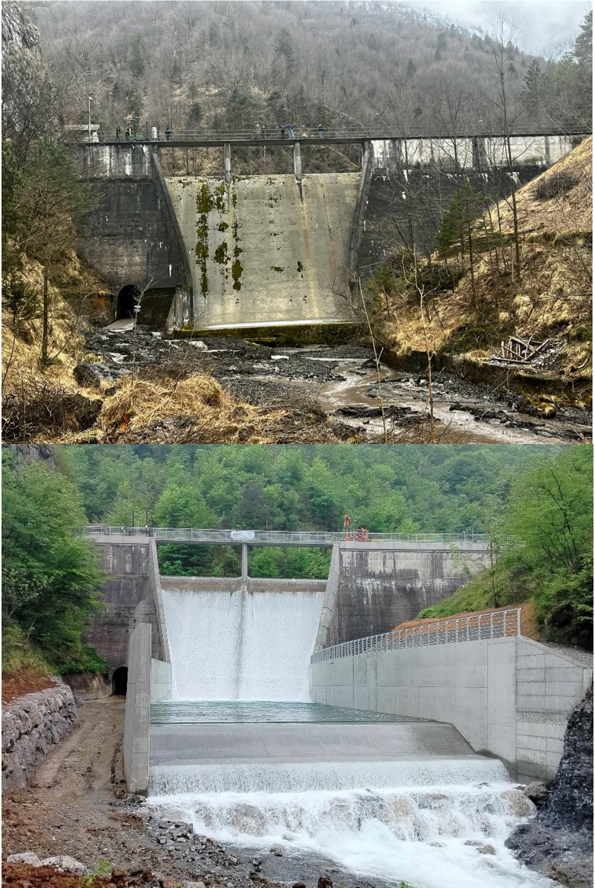
Figure 1 – Cassiglio dam before (upper image) and after (below image) the works
