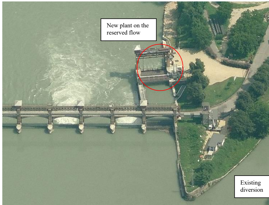
Figure 4 – Ecological flow plant built in the old ship lock at Chievo Dam, on the Adige River, just outside the city of Verona. The headrace channel of the main plant (located in the centre of Verona) is located on the right side of the river.
