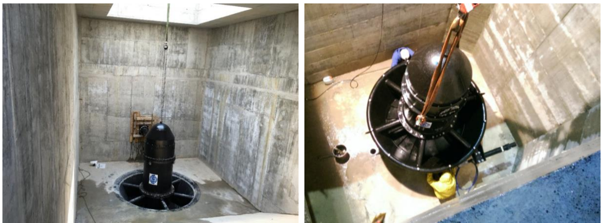
Figure 3 – Roggia Vetra (left) and Capriolo (right) PMG generator
